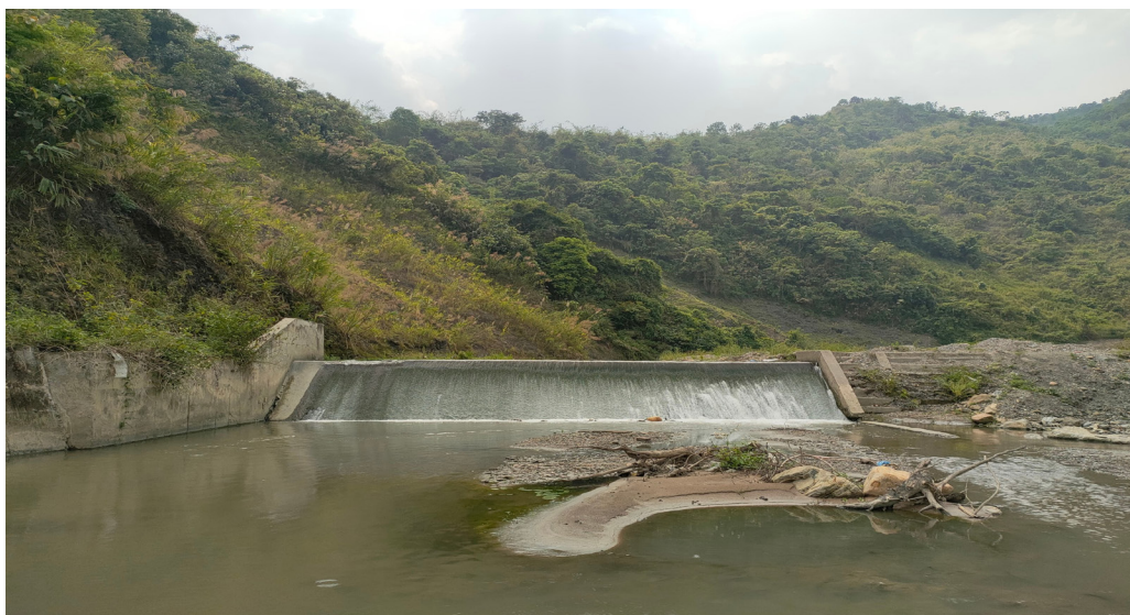
Figure 2. View of Na Muon check dam from downstream (taken in May 2022).
