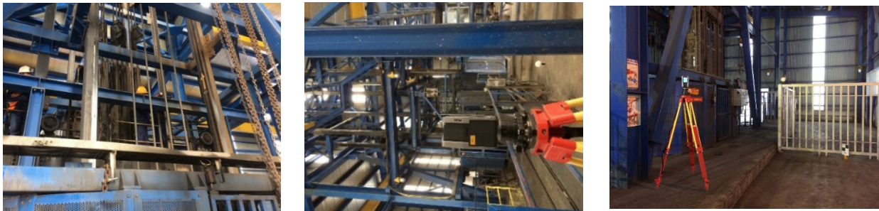
Figure 8. Columns and beams in the headframe of the mine shaft.
