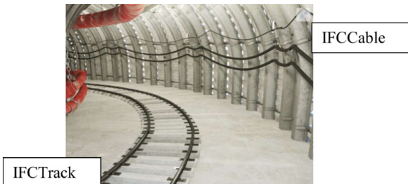
Figure 13. IFC of entities in tunnels.
